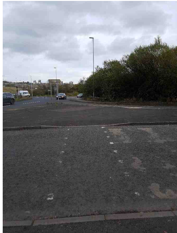
F.27 – Crossing facilities at the Banesley Lane Arm of Lamesley Roundabout
