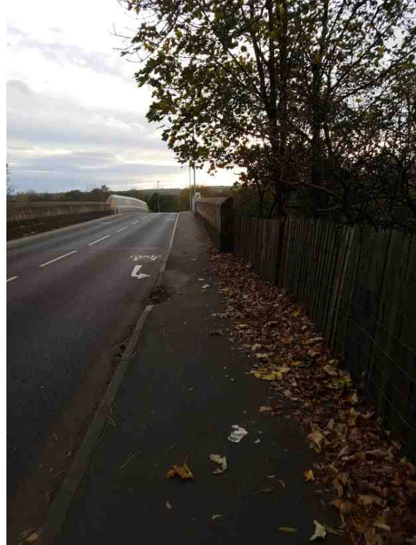
F.25 – South-westerly for Chowdene Bank Bridge
